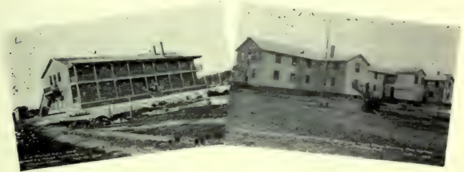
Hydro Development Plant, Whirlpool Rapids, Niagara.
